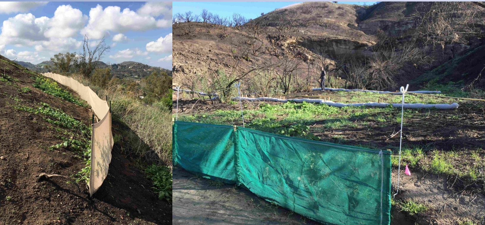
EXHIBIT 1: Typical EvoGuard (FKA: SOXfence®) Installation (Source: SOX Erosion Solutions)
