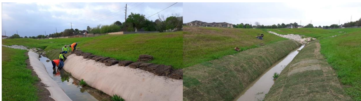
EXHIBIT 1: Typical DredgeSOX Installation (Source: SOXErosion)
